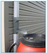
♦ Down Spout Diverters (Optional) The rainwater diverter is installed directly to the down spout to direct water onto your rain barrel. In the winter or when your barrel is full the diverter arm can be closed and the diverter becomes part of your down spout bypassing the collection system. The Diverter may be used with plastic or metal gutters and can be painted to match your down spouts.
